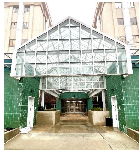
(back entrance to building on plaza parking)
